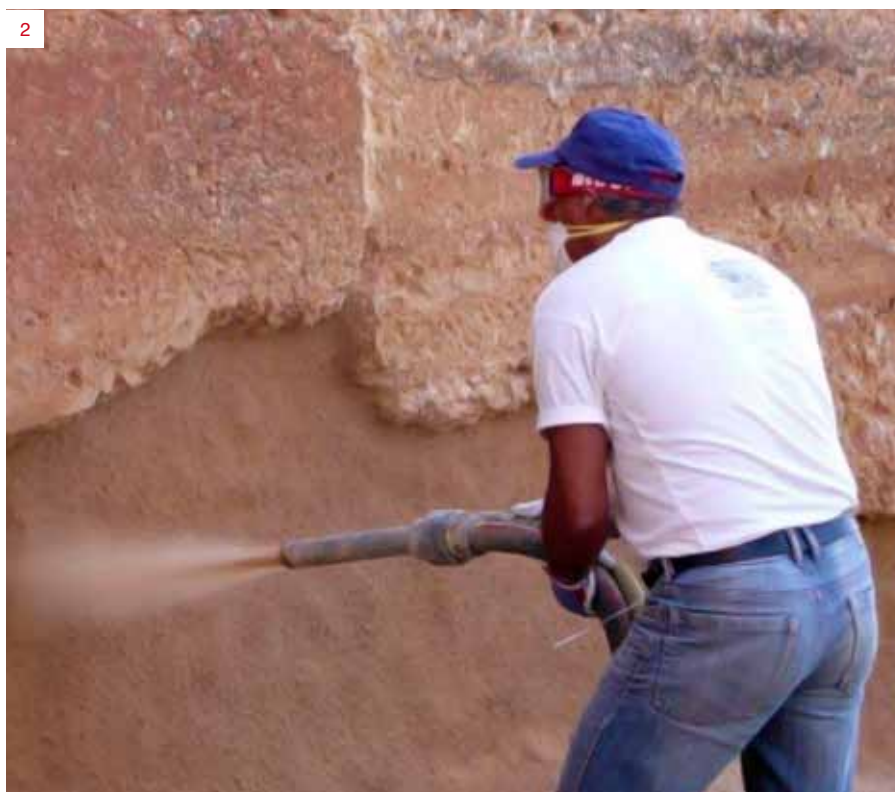
21 Sprayed earth: an innovative technique allowing for effective, durable and unexpensive rehabilitation of traditional raw earth constructions
